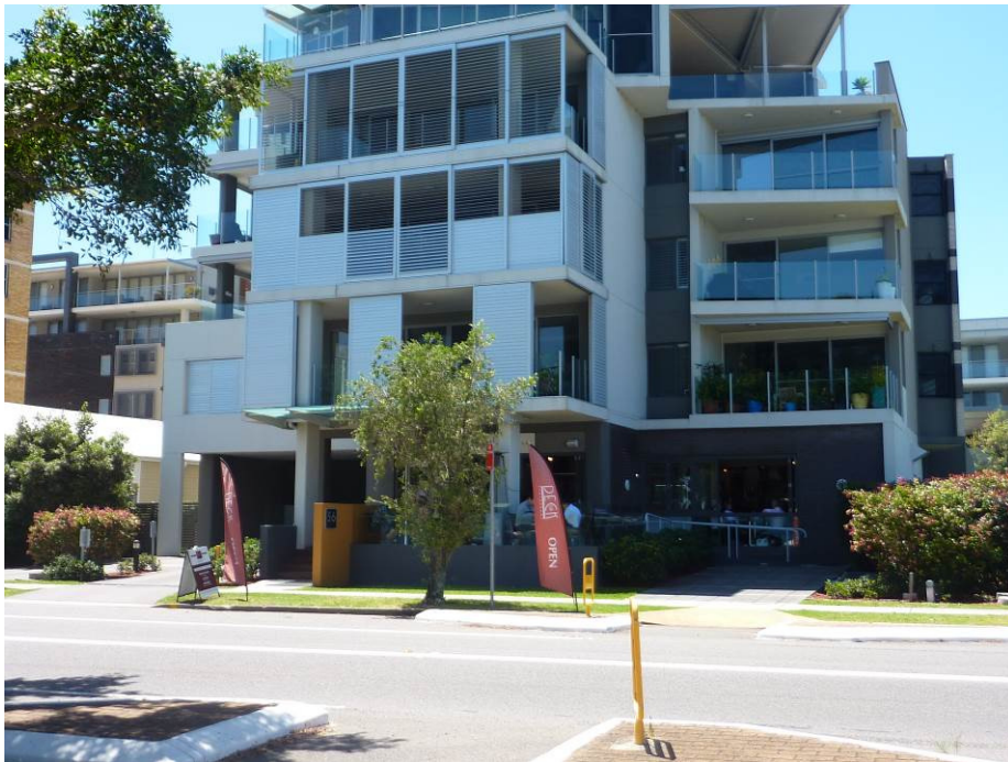
Deck Apartments on Brooks Pde with ground level café close to street
