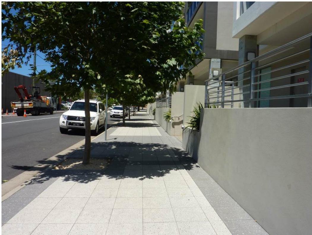
Wharf Apartments basement wall on Sharp Street
